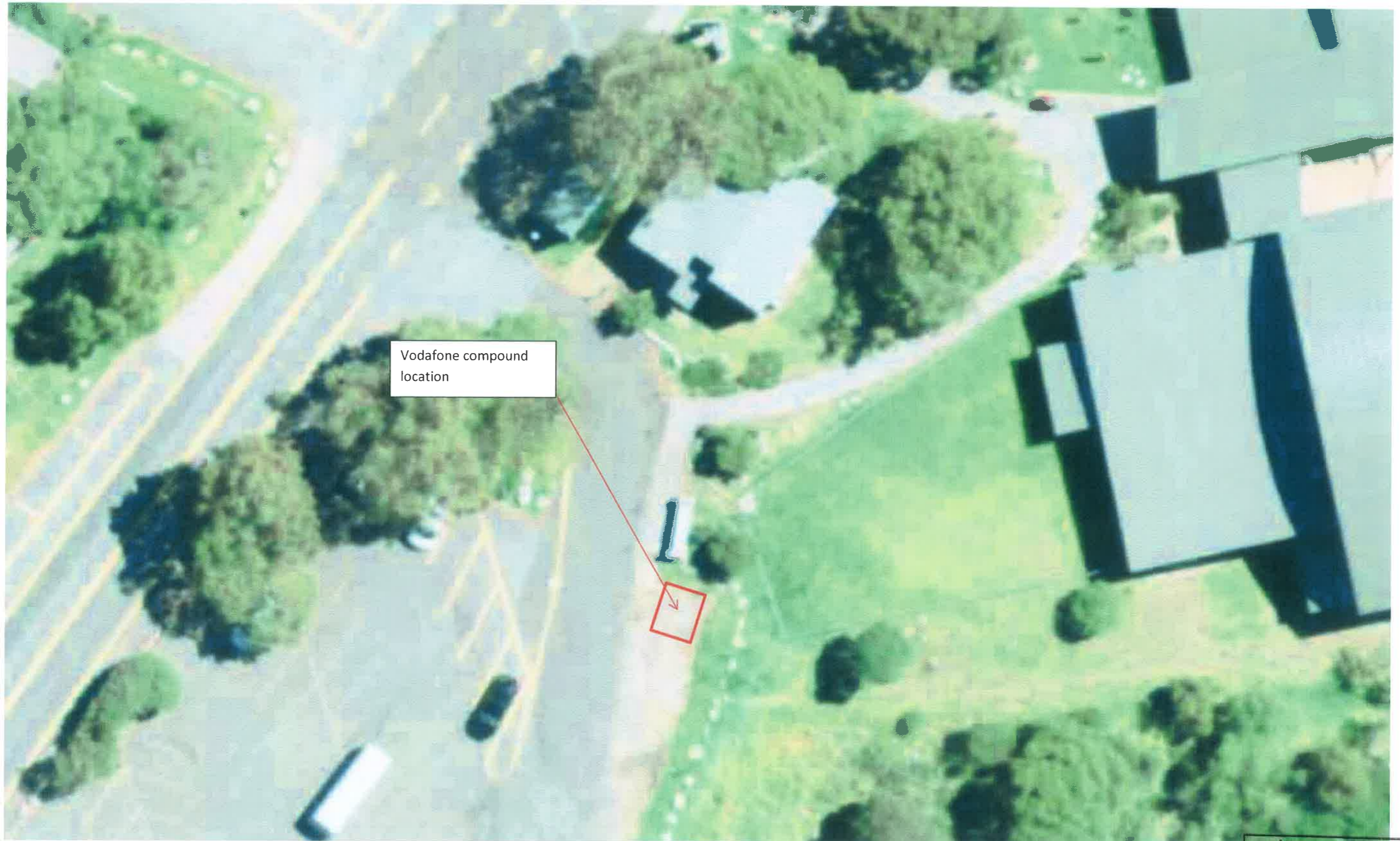
Vodafone Temporary Telecommunications Facility at Thredbo.
